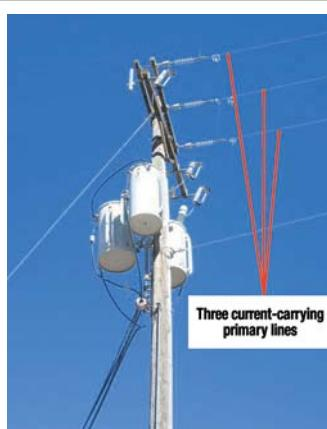
Balanced, three-phase system with three transformer cans
