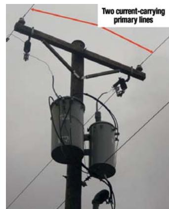
Unbalanced, three-phase system with two transformer cans, note the two different size transformers (50 and 25 kVA)
