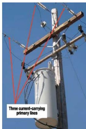
Balanced, three-phase system with a single transformer can
