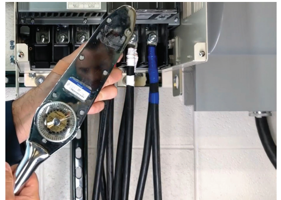
Figure 1: Proper torquing of power wiring done by a certified installer is one of the steps that help the drive's lifespan and increase ROI.
