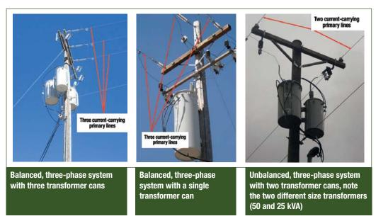
imbalance is transferred to the VFD. Therefore, when installing VFDs or other three-phase loads on open-delta supplies, proper steps must be followed.
