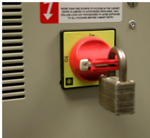
Fig 1.6 Disconnect Handle Positions – Shown OFF, With Padlock
