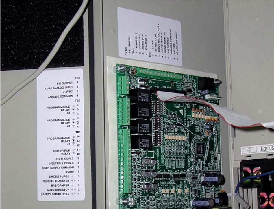
Fig 2.6 TB1 Control Terminal Locations, All Models
