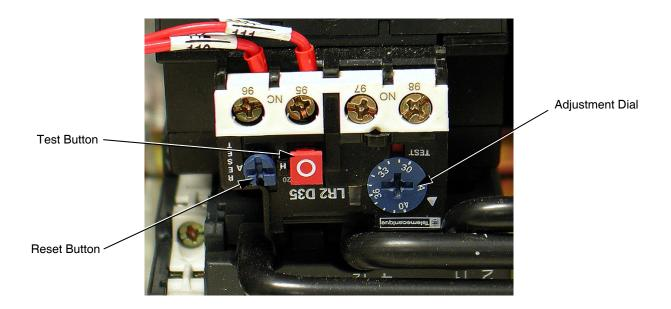
Fig 4.2 Overload Relay Detail
