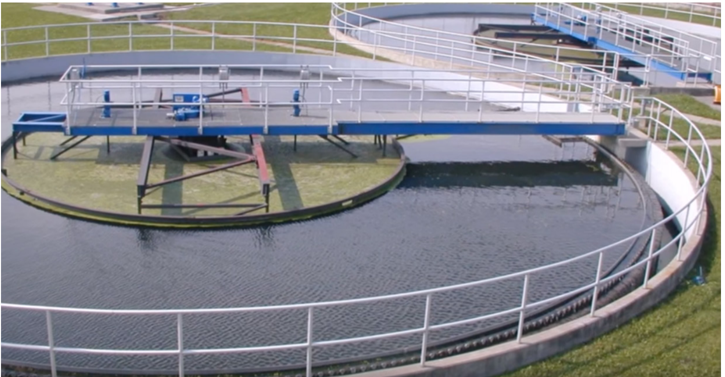
Retrofits to aging pump drives in water treatment facilities can produce significant efficiency improvements
