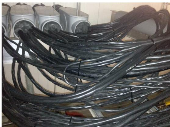
Extra wiring for multiple VFDs can lead to a lot of extra wiring and electrician hours
