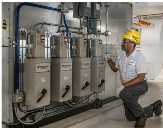
A VFD for each fan in an array requires sufficient mounting space
